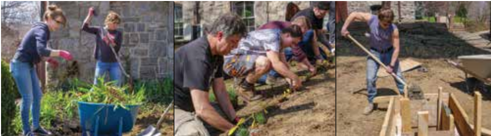
Water and Environmental Technology students designed and built a demonstration rain garden behind the Mellor Building. To reduce an estimated annual 50,000 gallons of storm water runoff, they removed non-native plants, regraded the site, and planted native vegetation. This project was supported by an Environmental Education Grant from the Pennsylvania Dept. of Environmental Protection, the Lancaster County Conservancy Water Week Grant Program, and Lancaster City.
